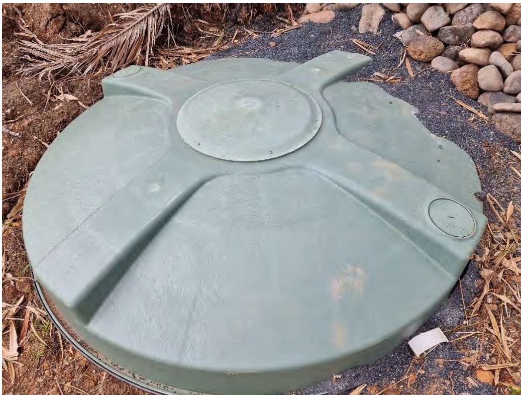
Plate 2.5 Existing primary septic tank which is performing satisfactorily (no leaks/seepage, odours or mechanical issues) and is sized appropriately for the dwelling
